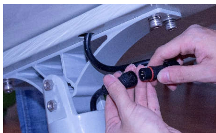
5.Lock the quadripuntal connectors of the Solar Panel & Horizontal Bracket together
