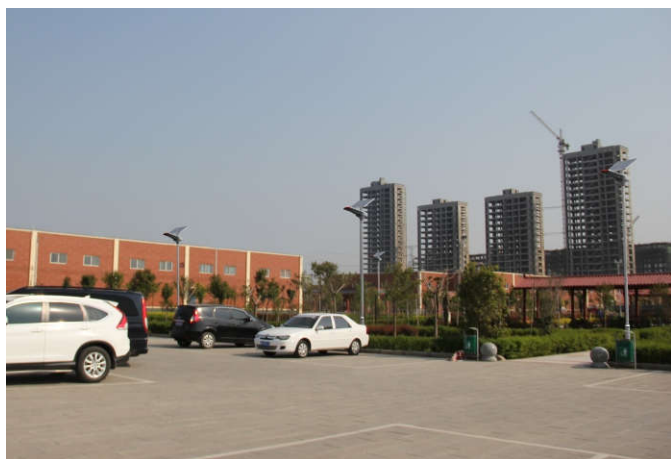
Open Parking Lot Lighting
