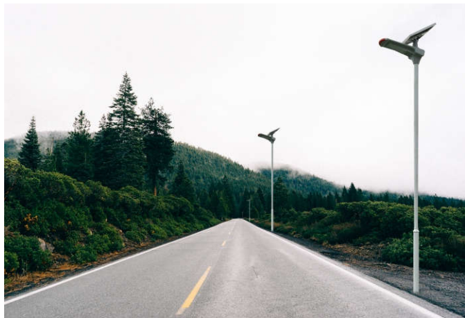
Traffic Road Lighting
